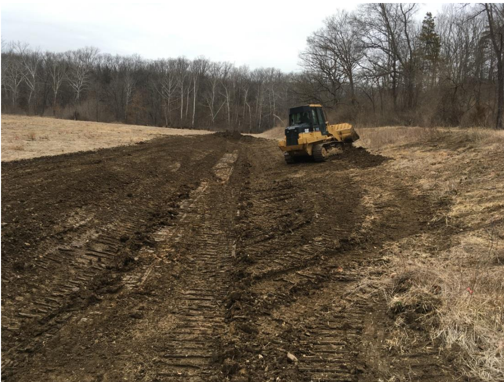
Figure 6. Stormwater swale during construction 2/13/2018
