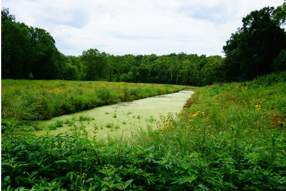
Figure 7. Stormwater swale summer 2020 7/20/2020
