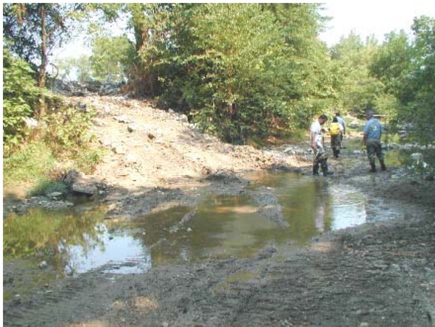
Photo 4. City of Columbia sewer line upgrade
