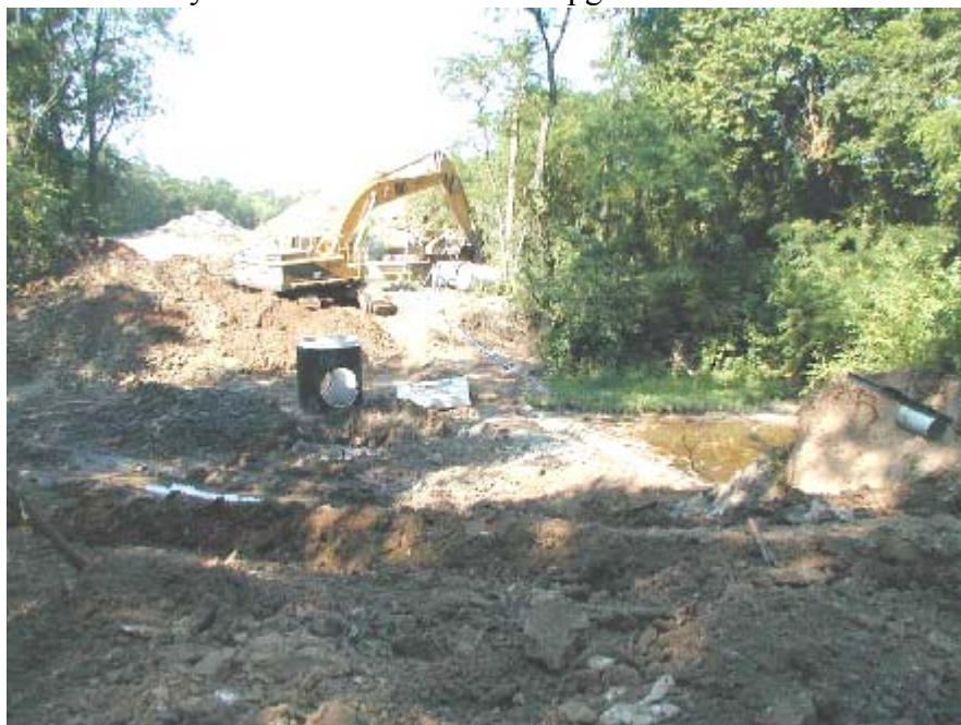
Photo 5. City of Columbia sewer line upgrade
