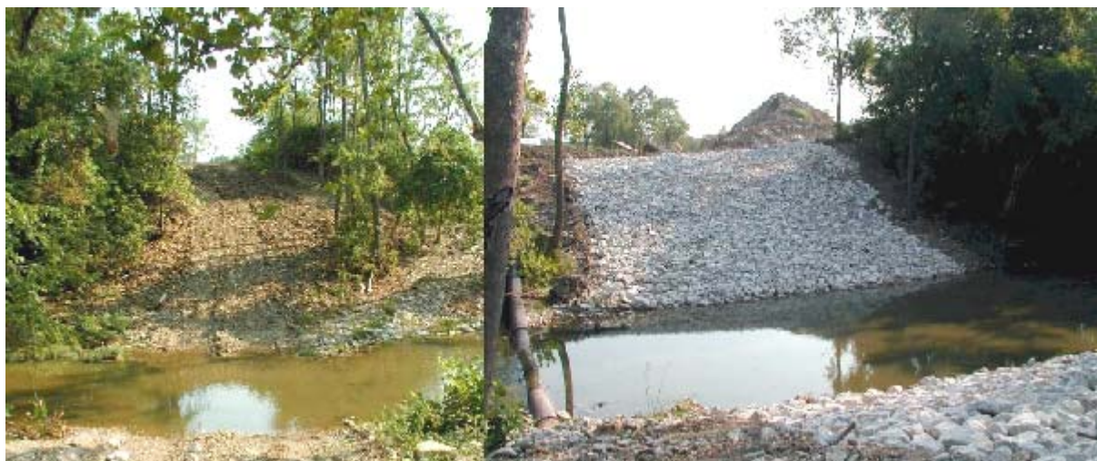
Photo 6. City of Columbia sewer line upgrade
