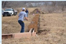
Laying out the Level Spreader
