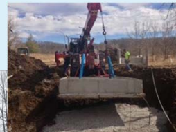
Setting the Diverter
