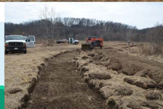
Cutting the Swale
