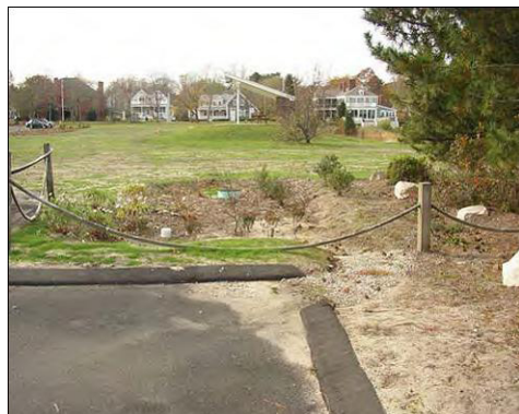
Figure 5.5 Dry Pond Treatment Area
