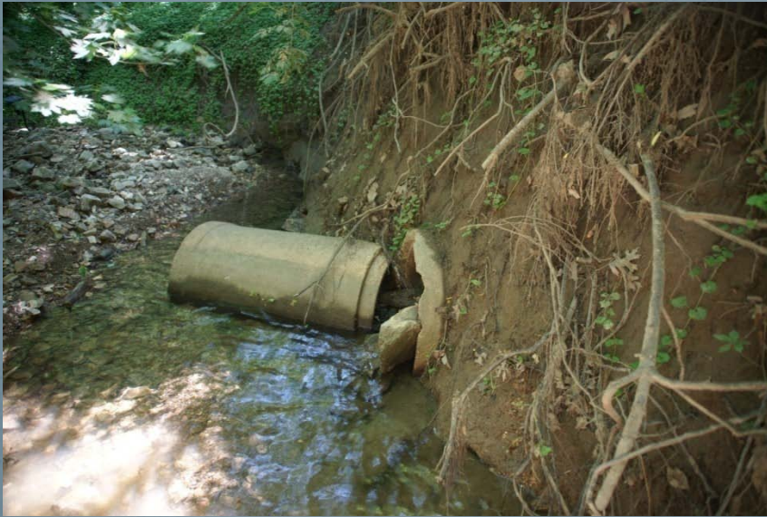
Cracked pipe
