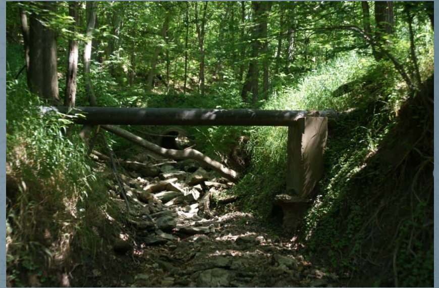
Old pipe crossing
