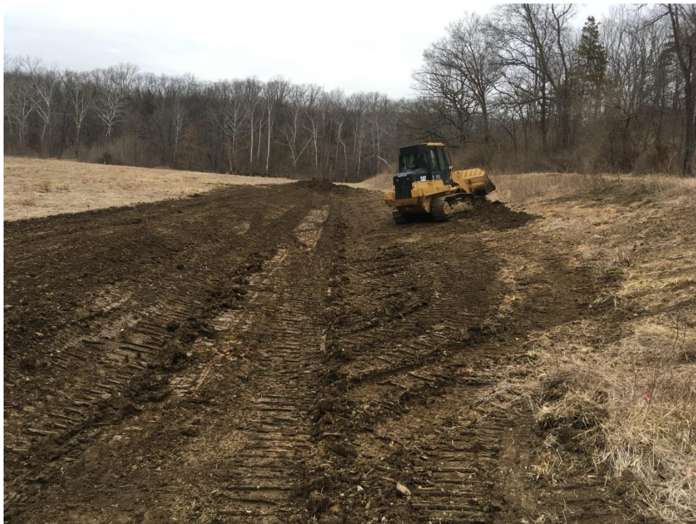
Stormwater swale during construction
