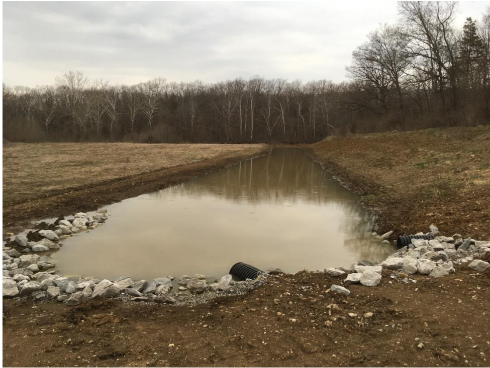
Stormwater swale post construction after rainfall event
